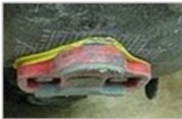
Figure 7b; Cleat Wedges fitted
